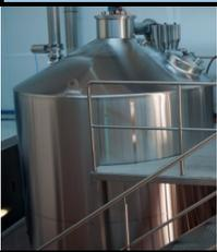
A beverage processing facility was installing a new processing tank to help increase production. After the tank had been installed, but before it was put into use, the tank was decontaminated with chlorine dioxide gas in order to make it safe for product to be introduced. Treatment time to complete the decontamination was under 6 hours and the tank went into use the next morning. No rinse or wash down was necessary as ClorDiSys' chlorine dioxide gas does not leave a residue.
